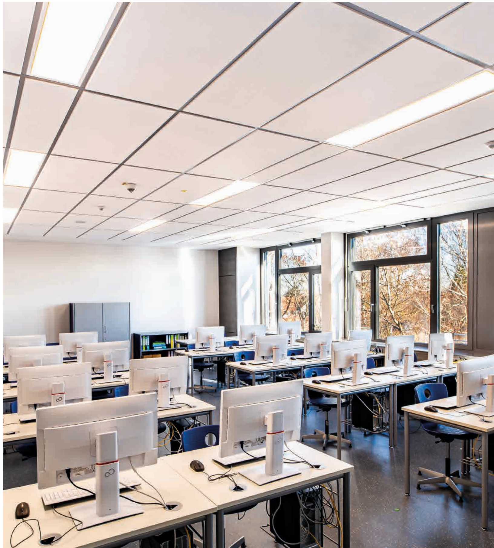
Sinfonia mineral ceiling, system S.3, T24 exposed profile, black Secondary school, Dachau, Germany
