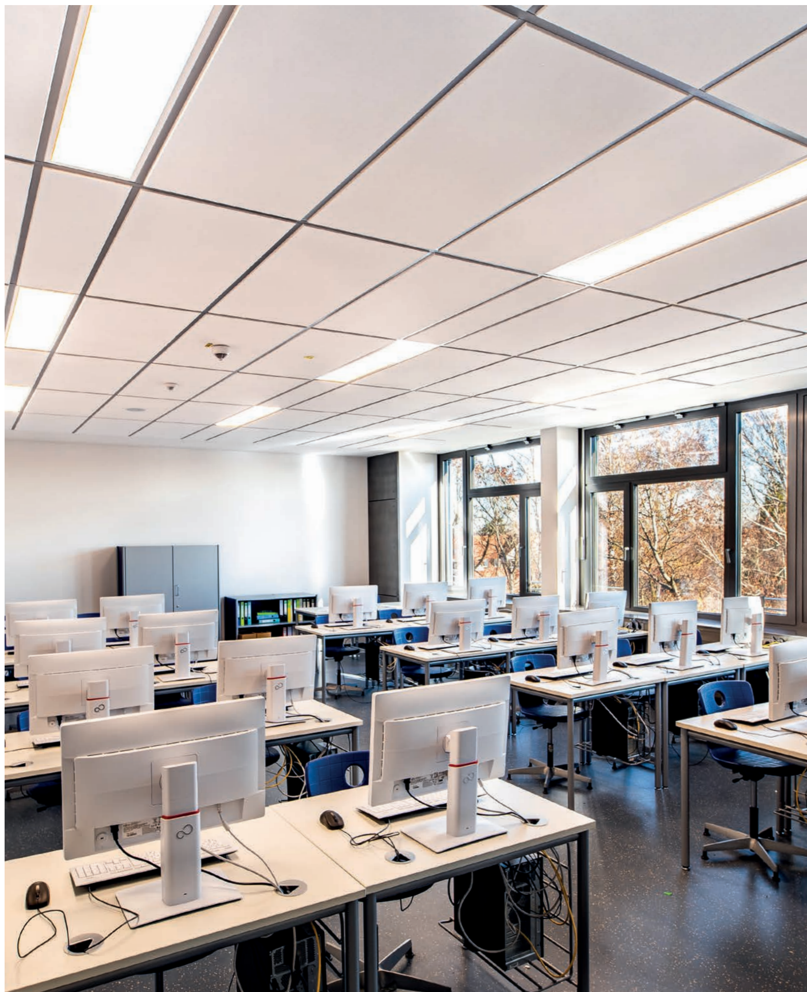
Sinfonia mineral ceiling, system S 3, T24 exposed profile, black Secondary school, Dachau, Germany
