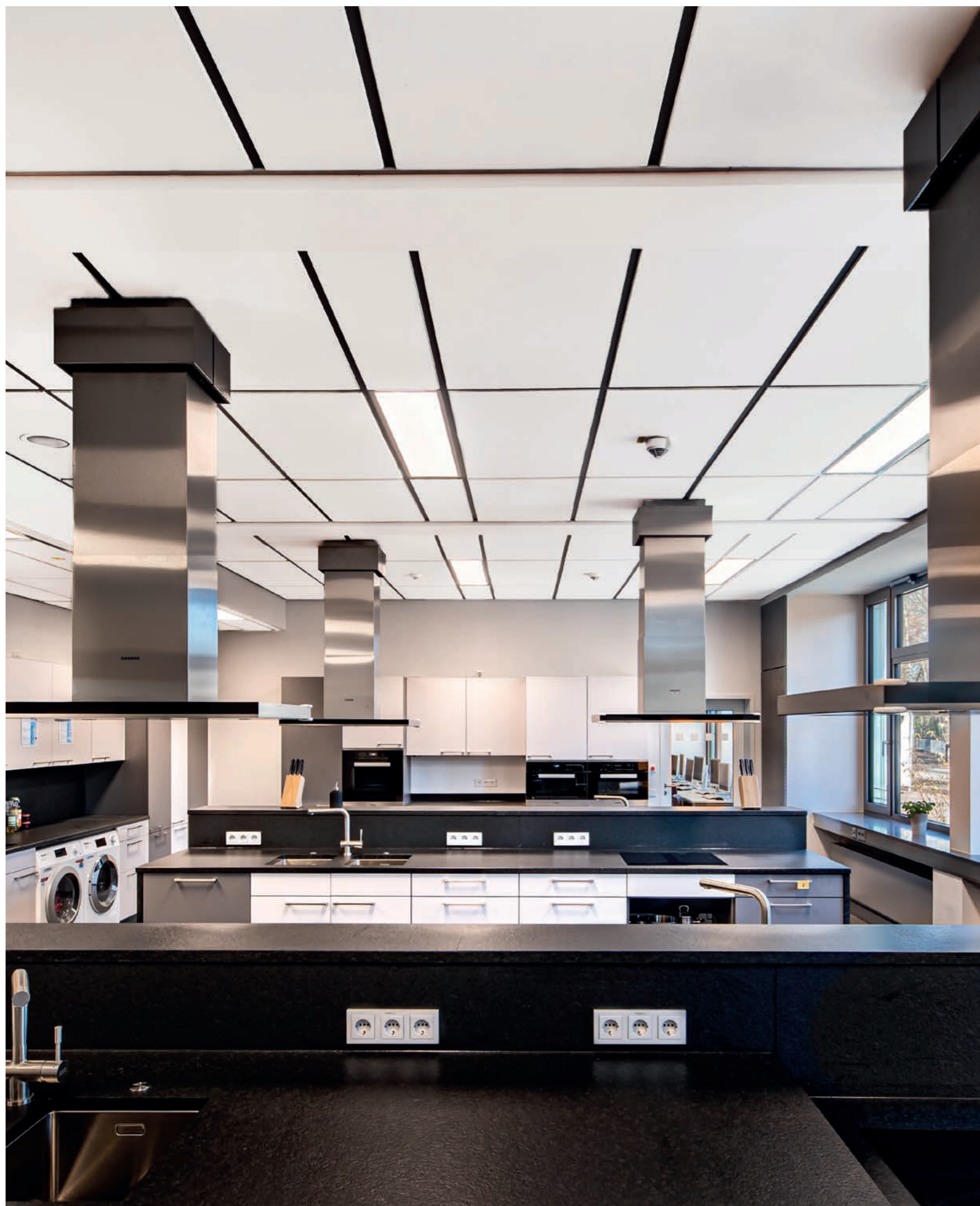
Humancare Sinfonia mineral ceiling, rectangular and square tiles, system S 3a, T24 exposed profile, black Secondary school, Dachau, Germany
